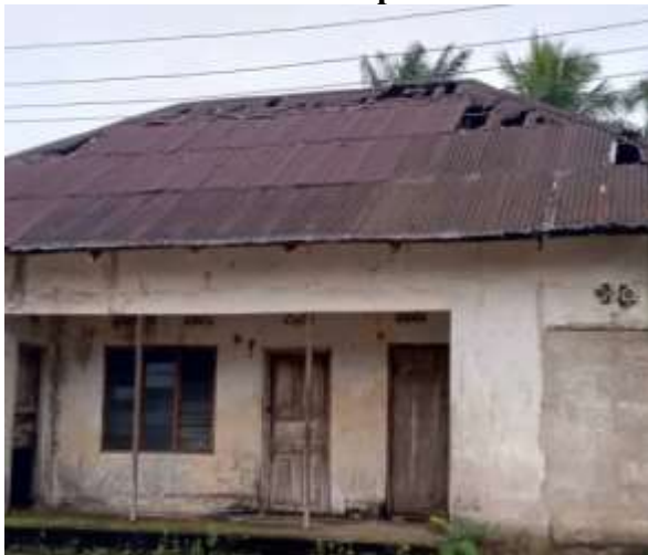
Plate 3: Perforated Zinc Roof
